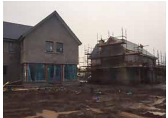
Phase 1 of ITC Douglas under construction
